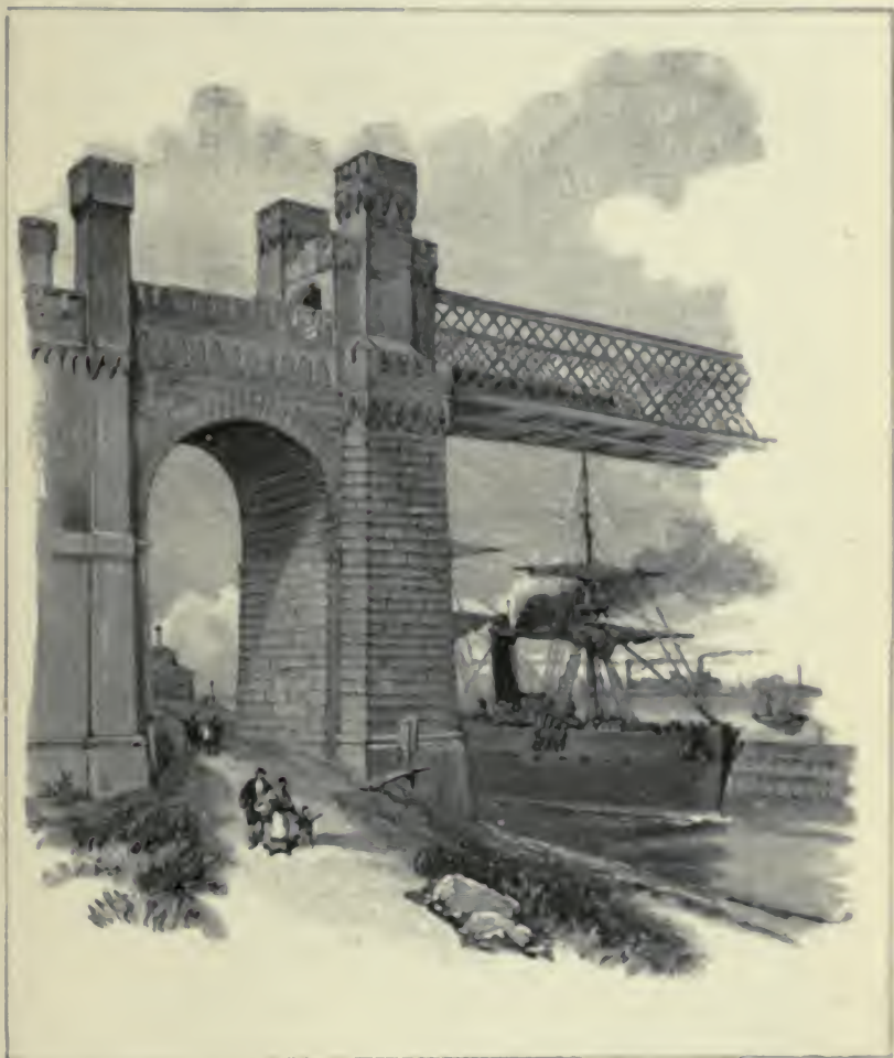
THE MANCHESTER SHIP CANAL: UNDER THE RUNCORN VIADUCT.
